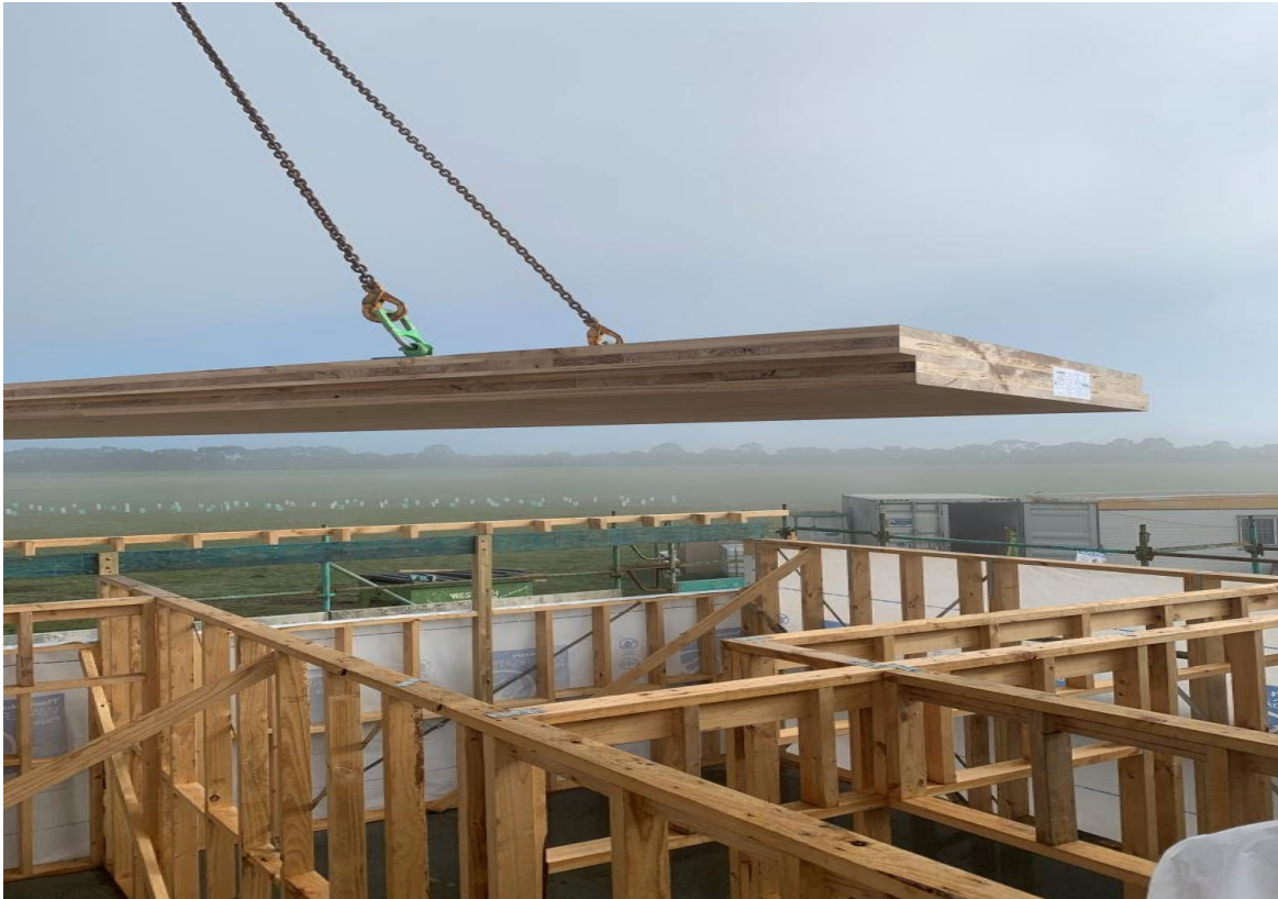
Figure 13: Cross laminated timber (CLT) panels manufactured by CLTP Tasmania from E. nitens for use in residential construction (Credit CLTP Tasmania)
